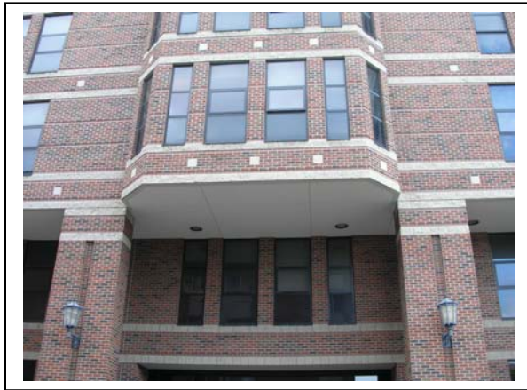
(Above) Reinforced masonry wall
